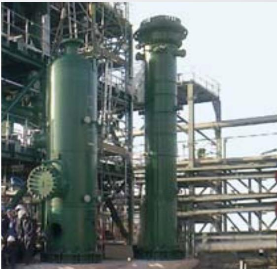
Figure 2 installed Twister Hydrate Separator for JT-LTX system
