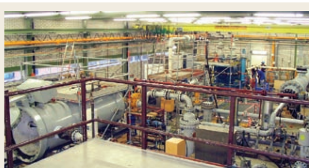
Fig. 5. Closed loop test facility (left: horizontal vessel containing tube. top: blue pump skid; right: water cooled HEX).
