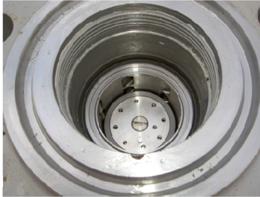
Figure 5: Change out of the valve trim to a SWIRL valve trim 14 Oct 2008
