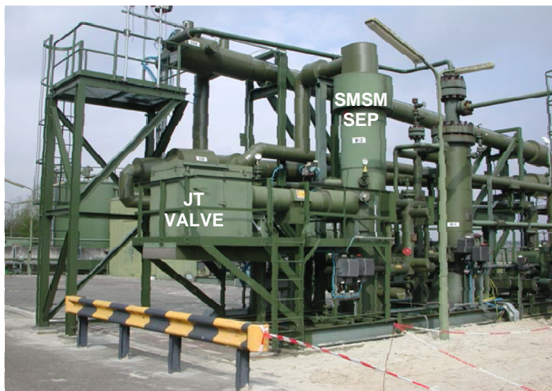
Figure 4: The NAM Opende Oost Gas Processing module
