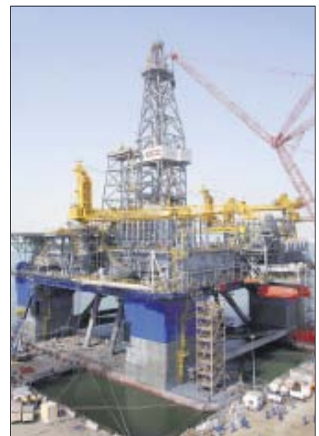
DELBA III during construction at GPC yards in Musaffah, Abu Dhabi.
